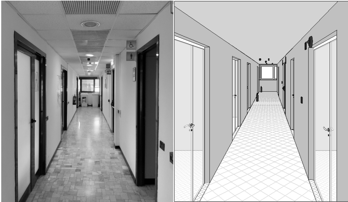
Figure 2. Camera sensors installed in the building corridor.
