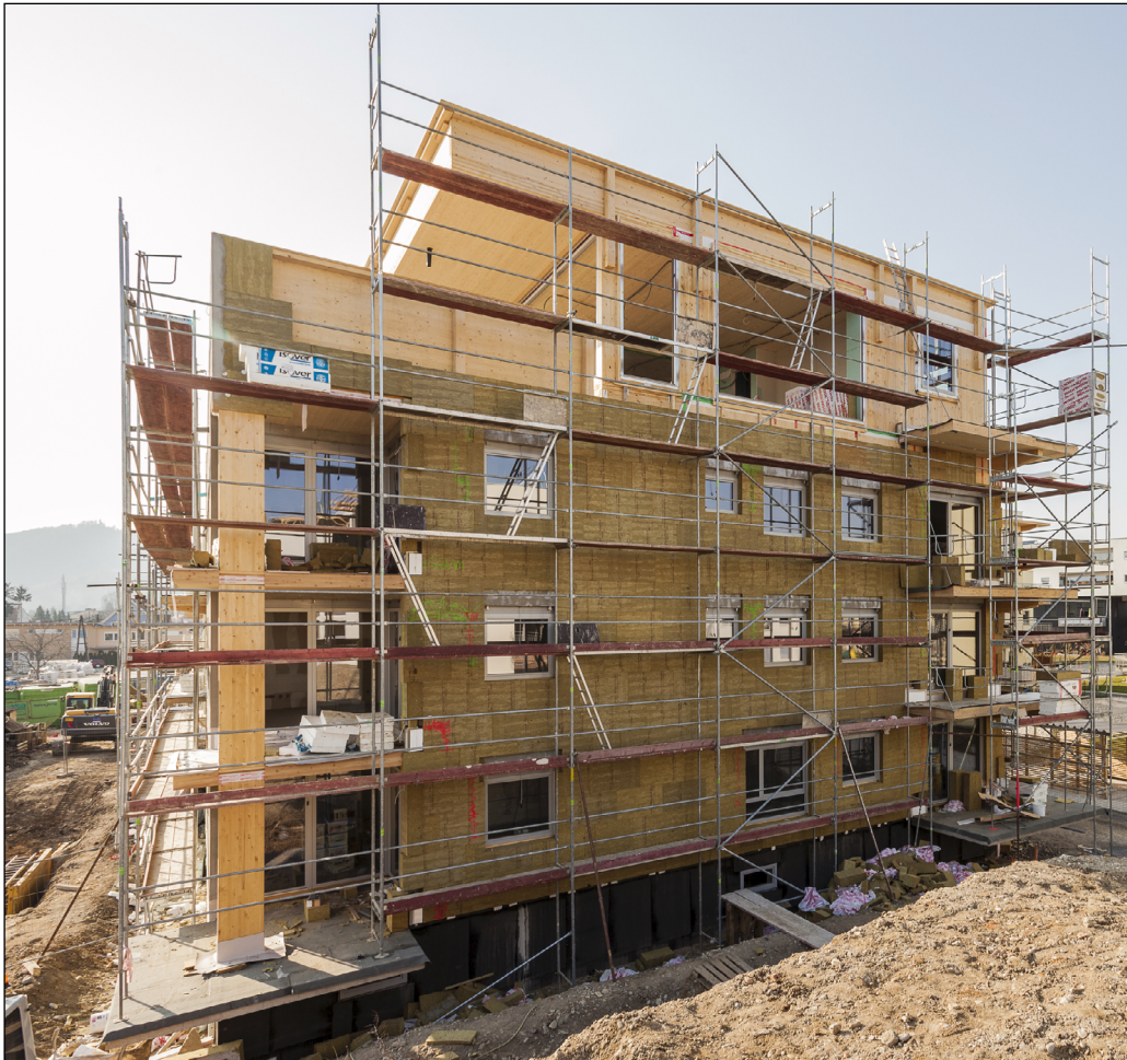
Figure 6: Case study building under construction. Source: Martin Grabner, TU Graz.
