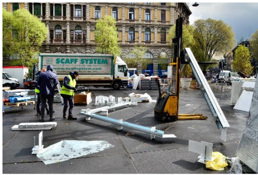
01 Assembling of primary beams of the roof structure
