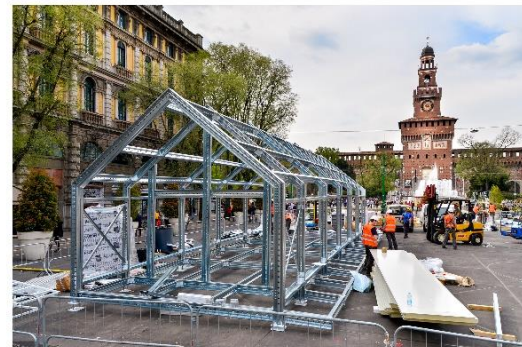
04 Overall view of the entire structure
