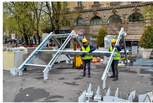
02 Assembling of the roof structure
