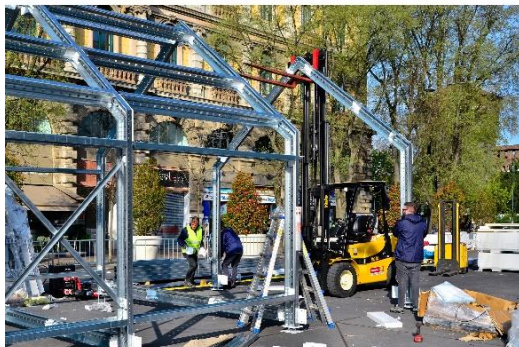
03 Completion of the structural modules
