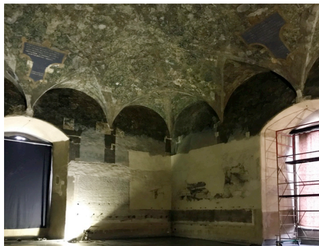
Figure 3: The Sala delle Asse after the restoration works, where the authors alternately obscured one of the two windows to check the light conditions.
