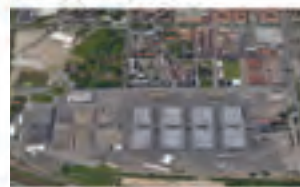
5 AREA EX MONTEDISON
