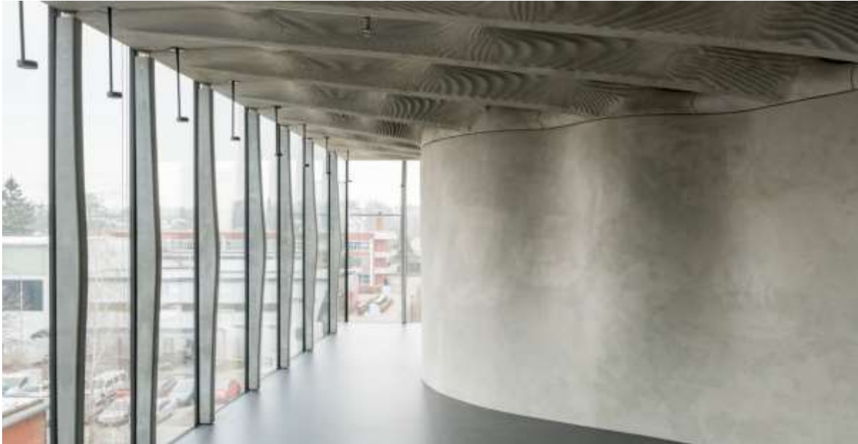
Figure 2. Concrete innovations on the first floor of the DFAB HOUSE: left , mullions produced with the Smart Dynamic Casting technology; right , Mesh Mould double curved wall; up , Smart Slab (photo: Roman Keller).
