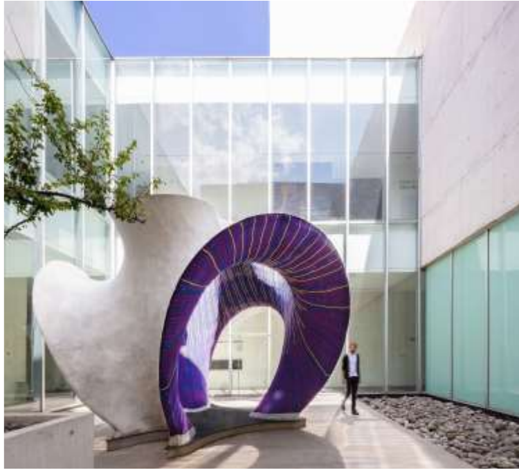
Figure 5. Finished KnitCandela concrete shell showing the soft textile interior and the smooth concrete exterior [96].
