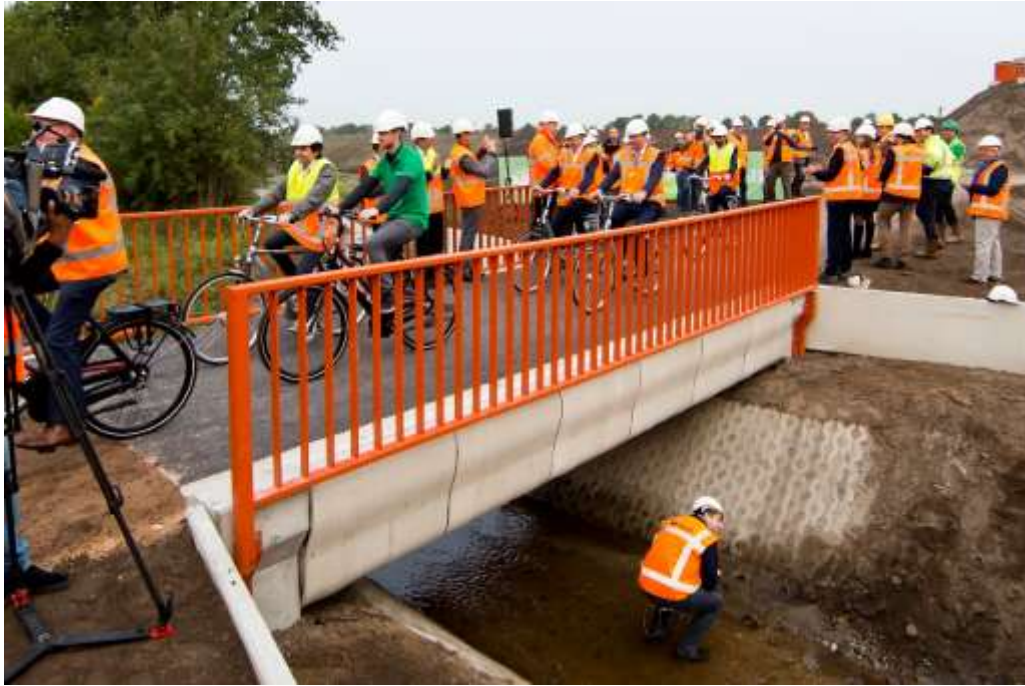
Figure 6: 3DCP bicycle bridge in Gemert, at the opening event in October 2017 (photo: Kuppens Fotografie)
