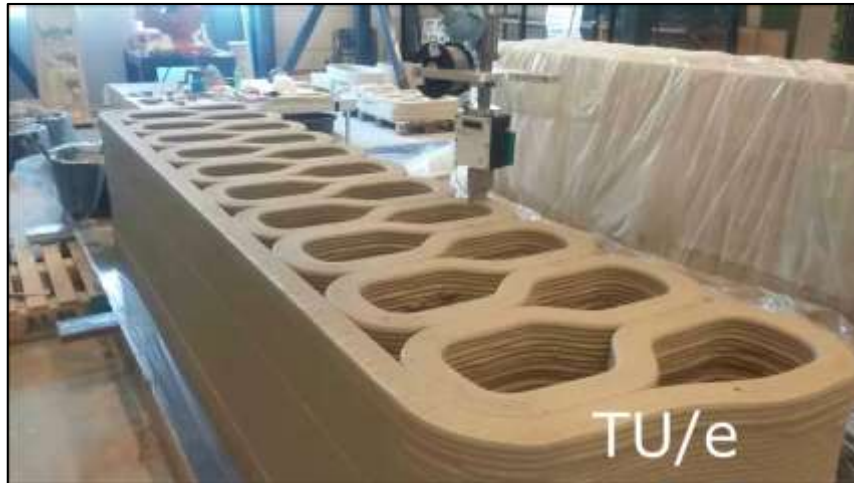
Figure 7: Printing of one of the parts of the bicycle bridge at the 3DCP facility of the TU/e
