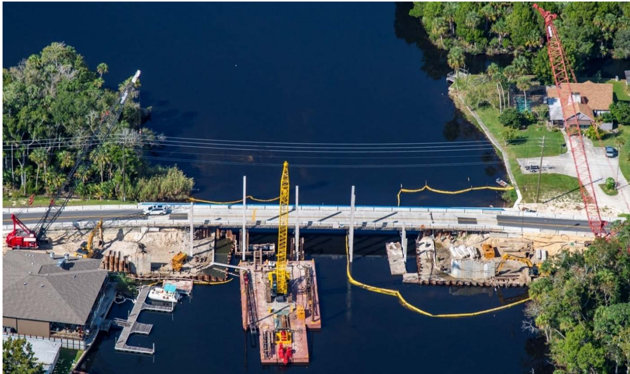
Figure 1 – Halls River Bridge aerial picture as of December 2018
