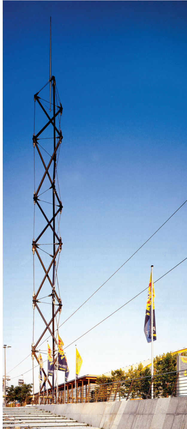
Figs. 5, 6 - Tensegrity T-prism; Gerkan, Marg und Partner (Architect) and Schlaich, Bergemann & Partner (Structural Design), Tensegrity Tower, Rostock, 2003 (H.G. Esch, Hennef-Stadt Blankenberg).
