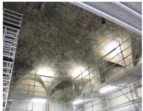
Figure 3: On-site photo of the current restoration works in Sala delle Asse
