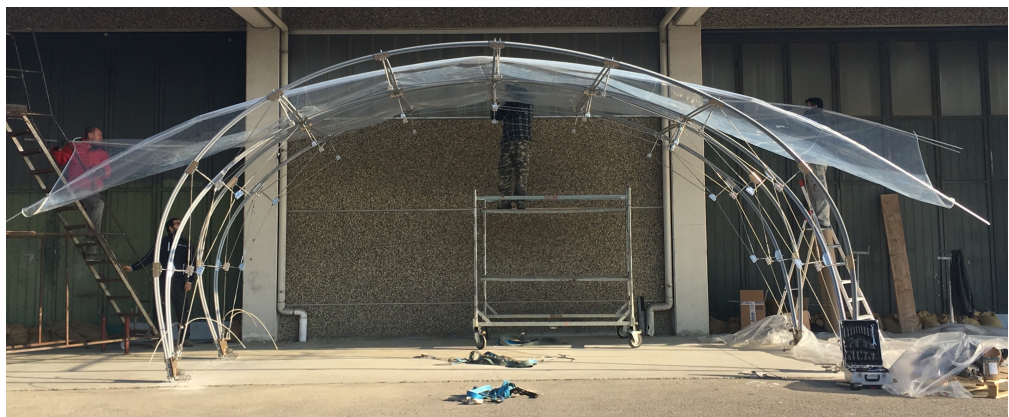
Figure 8. ETFE foil installation
