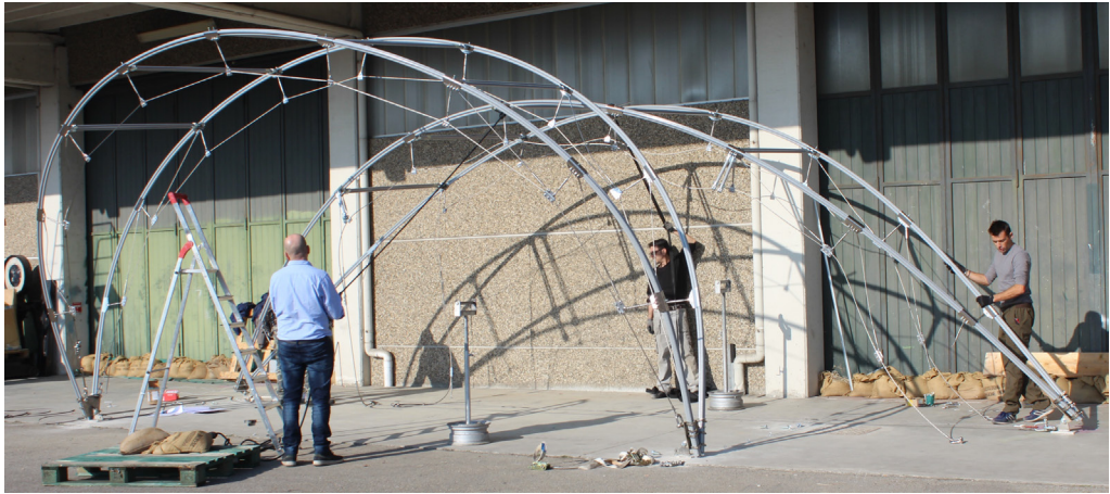
Figure 7. Second module erection during arches bending
