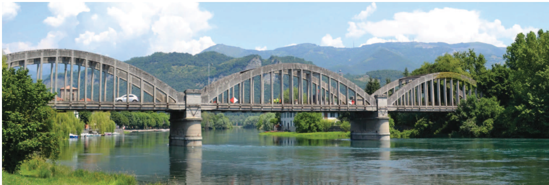
Figure 3: Present downstream view of three-span Brivio bridge (1917) on river Adda; Brivio (LC) right bank (left), Cisano Bergamasco (BG) left bank (right).
