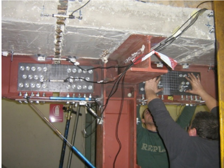
Figure 29 Repair operation after the full-scale tests
