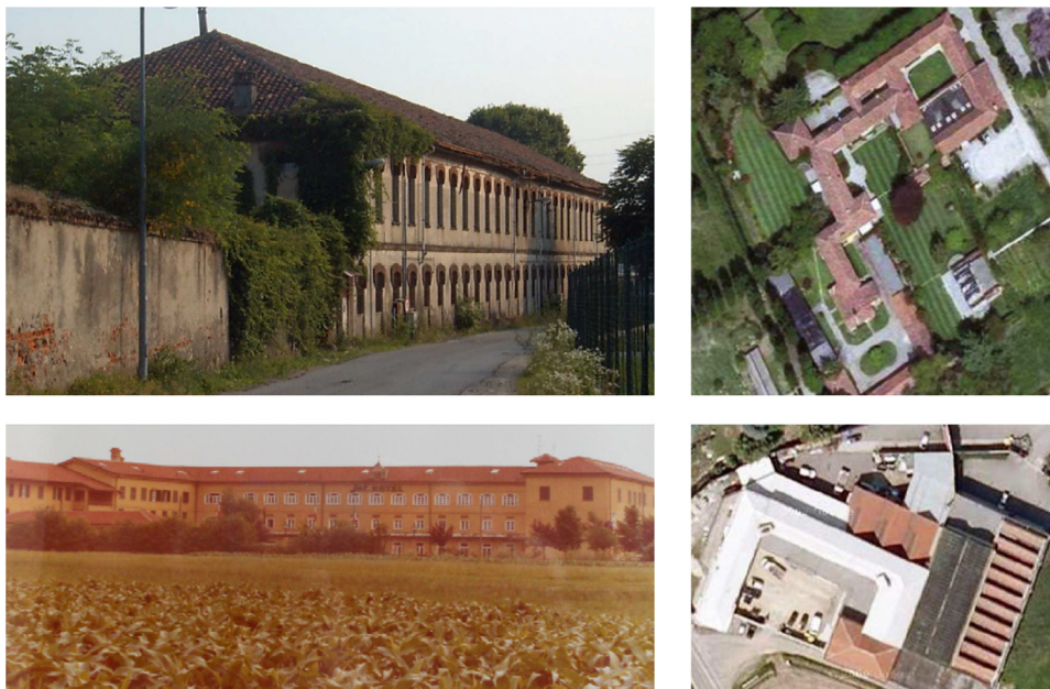
Fig. 2. Pictures of 4 former industrial buildings still existing (from the top left: silk factory Caudano; paper mill La Carignana; paper mill Belgrado; paper mill Montruca). Elaboration from [47].
