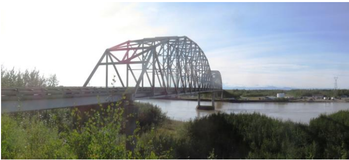
Figure 7. Picture of the bridge structure and the pier in the riverbed (photo credit: Don Moe, http://donmoe.com/blog/2016/01/15/fairbanks-ak-to-denali-highway/ ).
