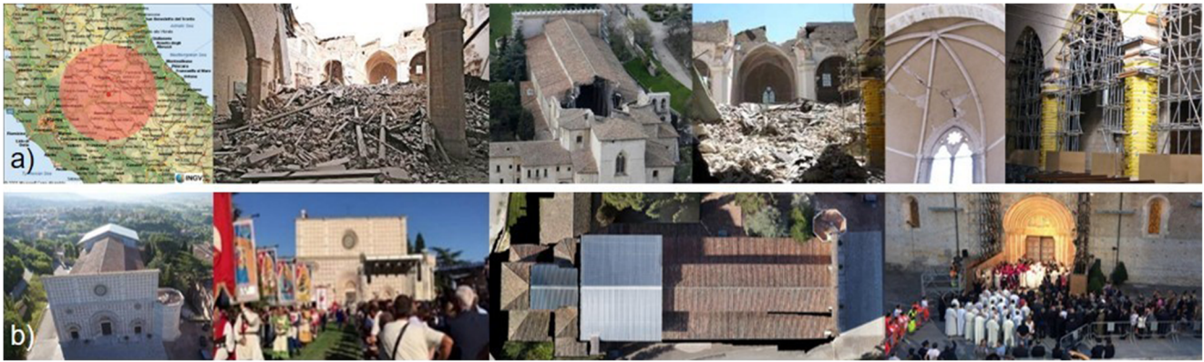
Fig. 1 Photographic sequence showing (a) the area stricken by the 6th April 2009 earthquake and the damages occurred to the Basilica and (b) the provisional covering realized after the seismic event and the opening of the Holy Door during the Jubilee Forgiveness procession
