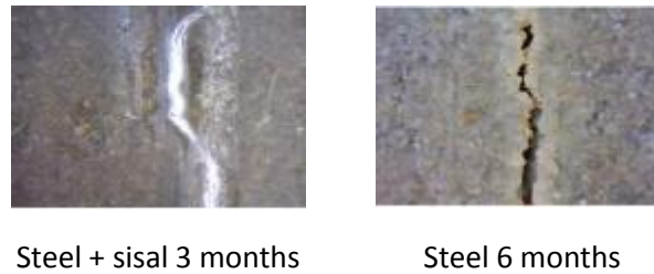
Figure 3. Comparison between crack healing in HPFRCC with steel+sisal fibers and steel only fibres subjected to wet and dry cycles. Specimens were pre-cracked at 2 months (0.5 mm crack opening). The bottom images show crack healing after 3 months curing in daily wet/dry cycles for the samples with steel and sisal fibres, and after 6 months curing for steel fibres only.
