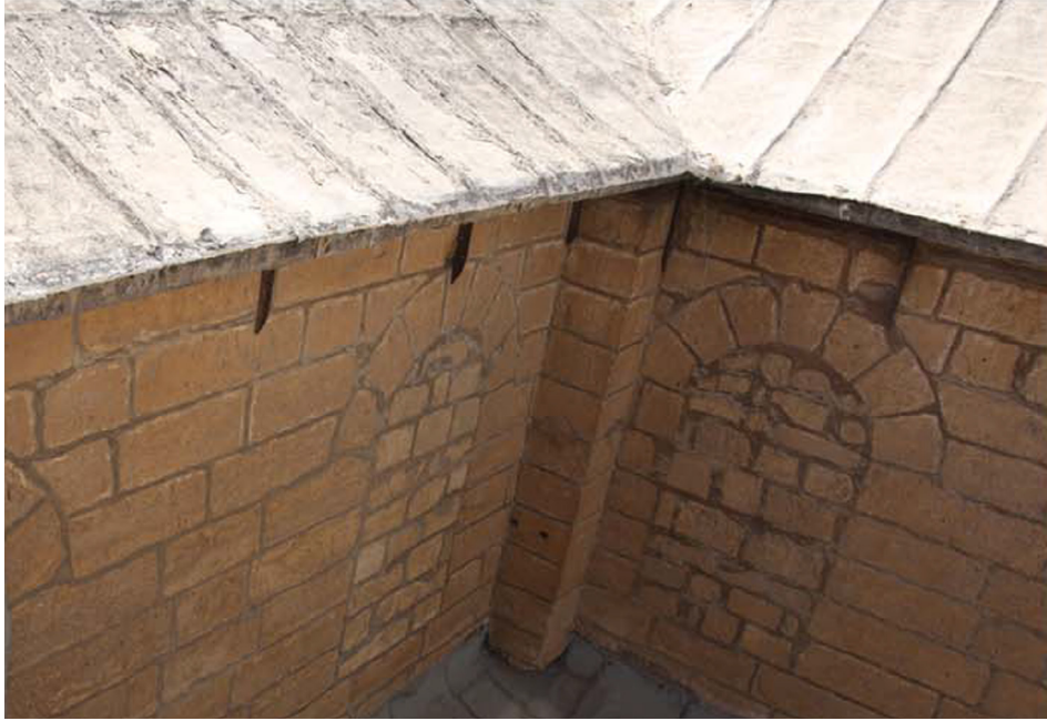
Fig. 16. Buffered windows at the intersection between the apse and transept.
