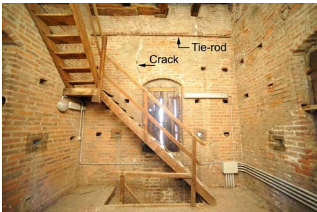
Fig. 4 Metallic tie-rod installed below the belfry (Level 2, West side)
