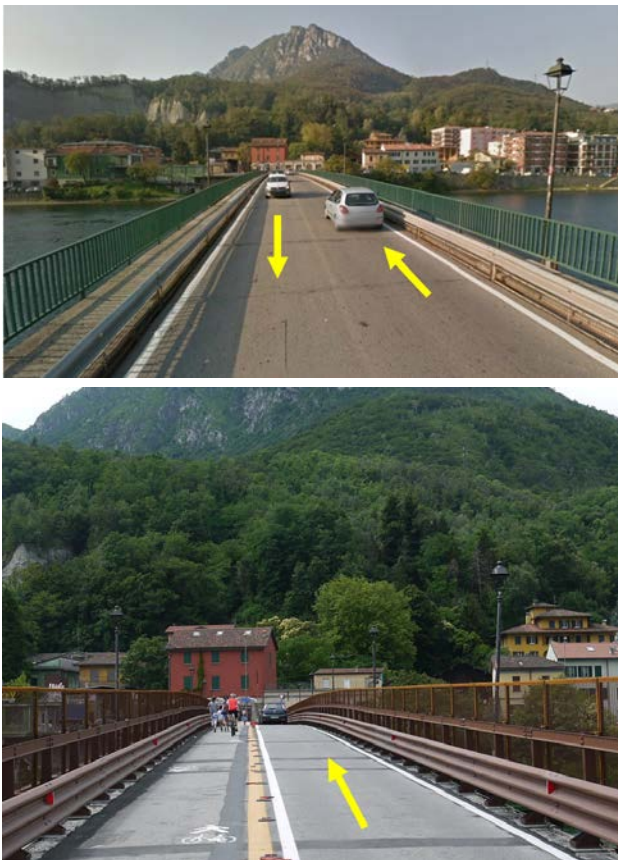
Figure 8. The bridge before and after the intervention: from two (top) to a single lane for cars (bottom), with a new pedestrian lane.
