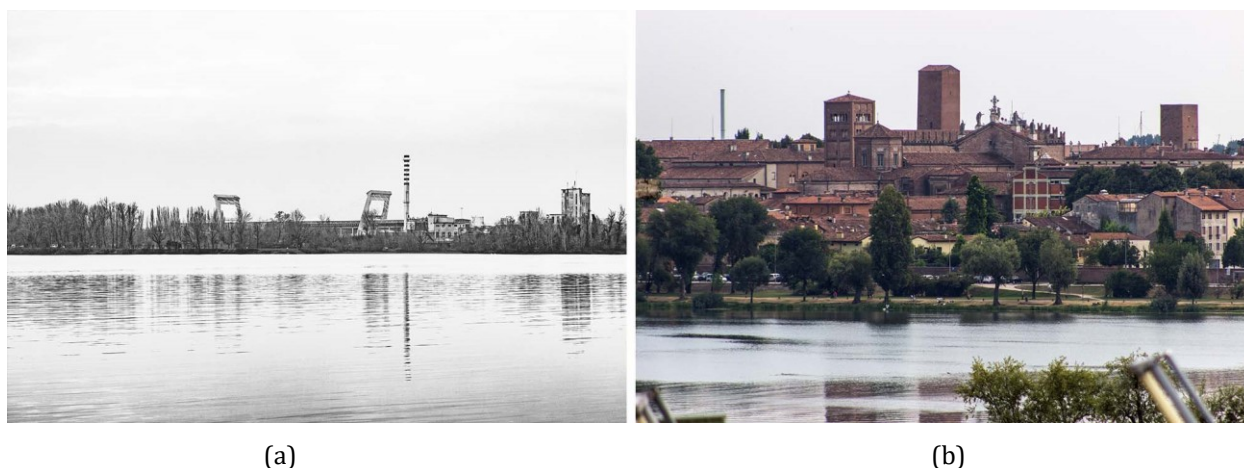
Figure 5: Visual relations. (a) Burgo Paper Mill seen from the Monumental City. (b) Monumental City seen from the Burgo Paper Mill. Source: D. Galli (2016), G. Sempredon (2016).
