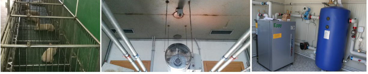
Fig. 3. The piglet room (left), the pre-existing gas burner (centre) and the new GSHP system (right).
