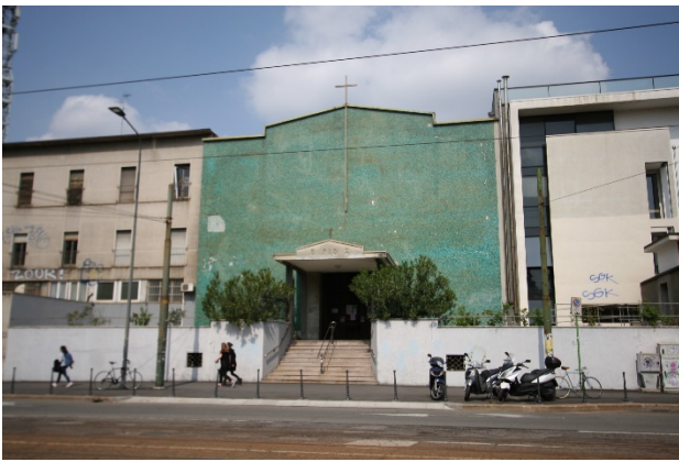
Figure 1 – The southern façade of St. Pio X Church (Case Study 1), facing Piazza Leonardo da Vinci square.
