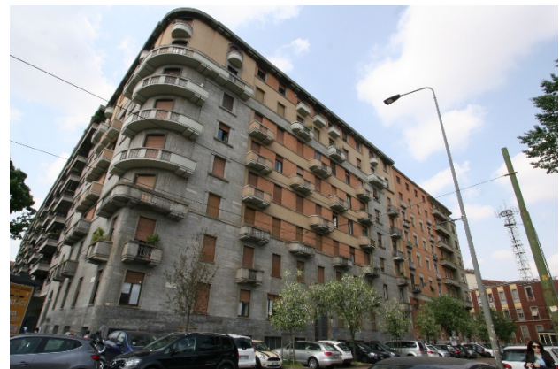
Figure 4 – Eastern façade of the residential building in Piazza Leonardo da Vinci square, Milano, Italy (Case Study 2).
