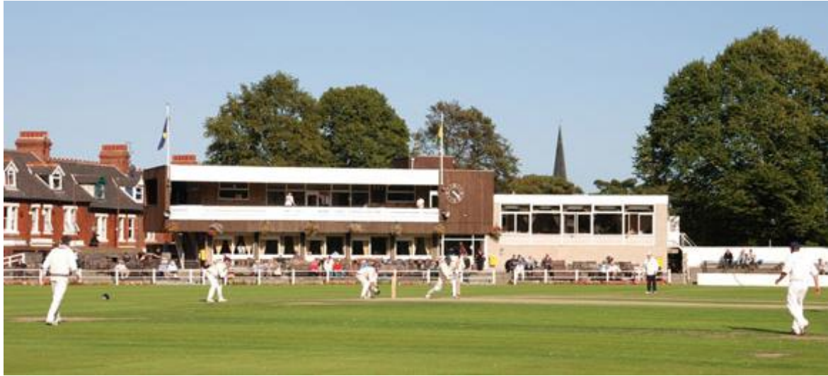
Figure 9. The pavilion by L. J. Couves & Partners at Jesmond Cricket Ground
