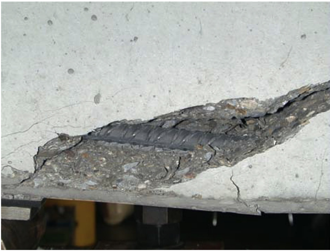
Fig. 9. Failure of beam T75L-NN: fracture of aggregates.
