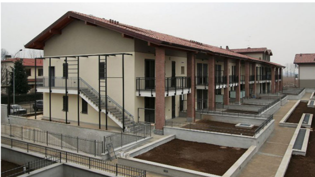
Fig. 4 View of the building no. 1
