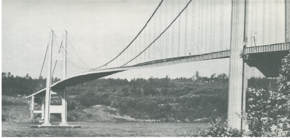
FIGURE 1. The collapsed Tacoma Narrows Bridge (1940).
